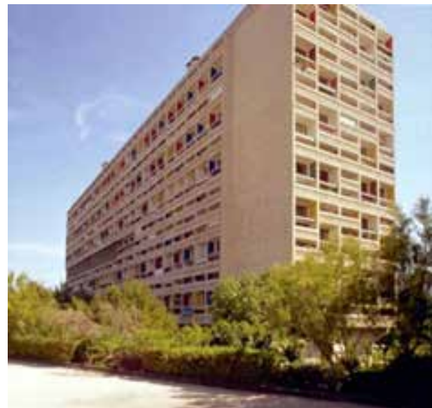
Figure 5.1.31 Marseille Housing Unit
