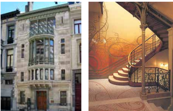
Figure 5.1.12 Exterior and interior views of Hôtel Tassel
