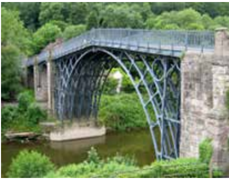
Figure 5.1.6 First metal bridge over River Seven
