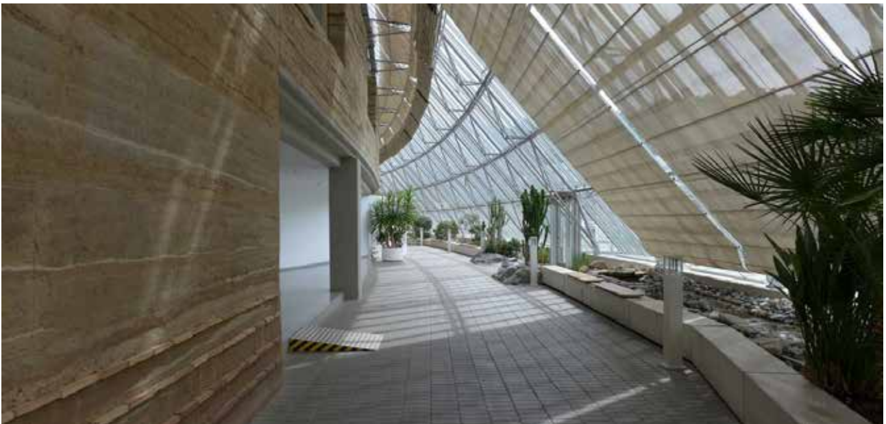
Figure 4.1.6 Hospital in Feldkirch, Vorarlberg, where clay is used for main bearing wall., photo: Veronika Kotradyová
