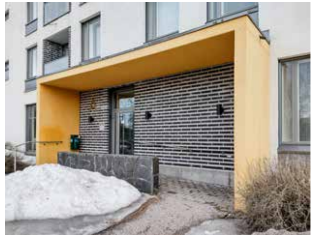
Figure 3.2.6 Example of projected entrance, Espoo – Helsinki (Čerešňová)
