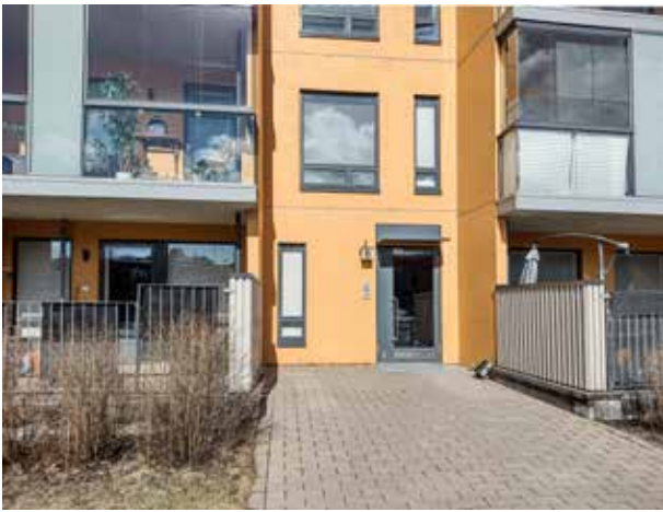
Figure 3.2.5 Example of flush entrance, Haso – Helsinki (Čerešňová)
